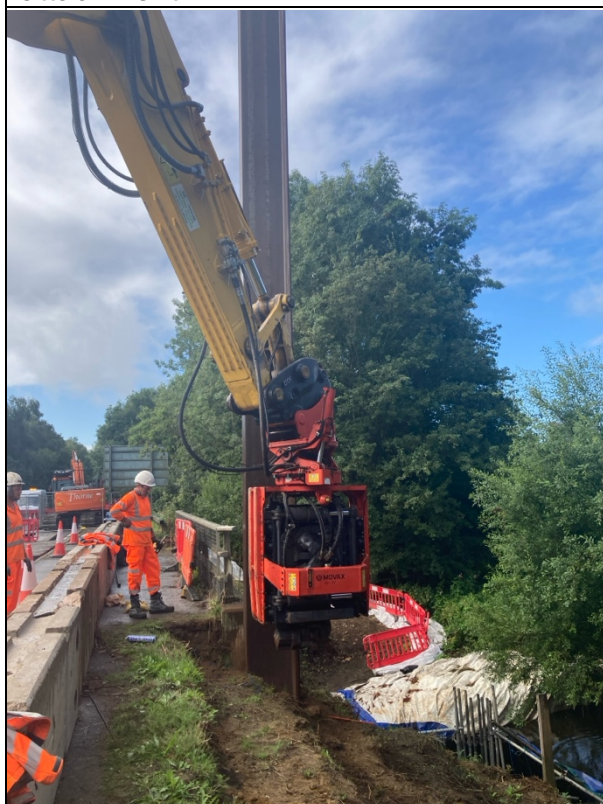
Figure 1: Back driving piles using DH25 attachment
