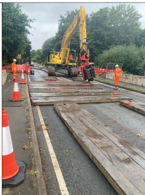
Figure 2: Bog mats laid out to avoid damage to the road
