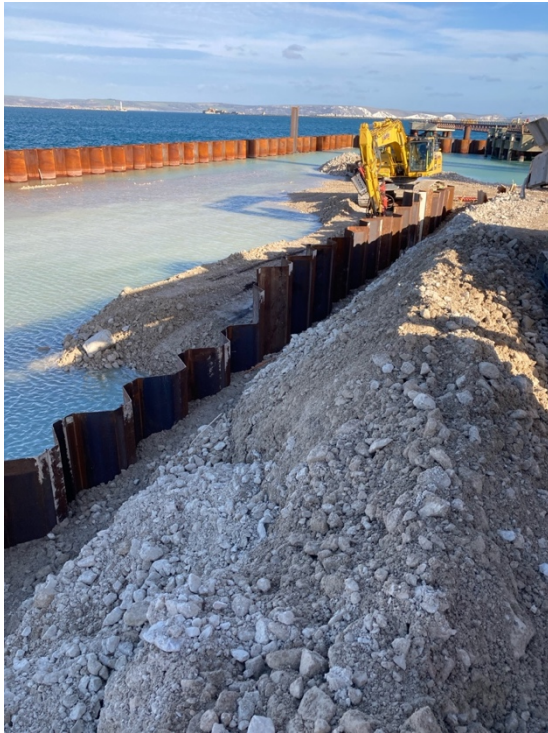
Figure 1: The sheet pile wall
