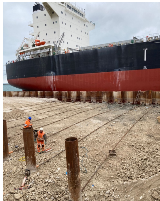
Figure 4: The sheet piles and tubular piles with the anchor rods between
